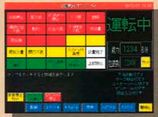
Operation Control Board with Graphic Indication
